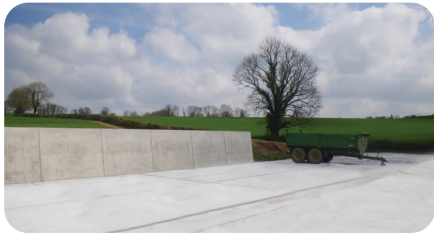
Agri Construction Project, Innishannon
