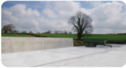
Agri Construction Project, Innishannon
