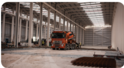
Large-Scale Logistics Warehouse, Little Island
